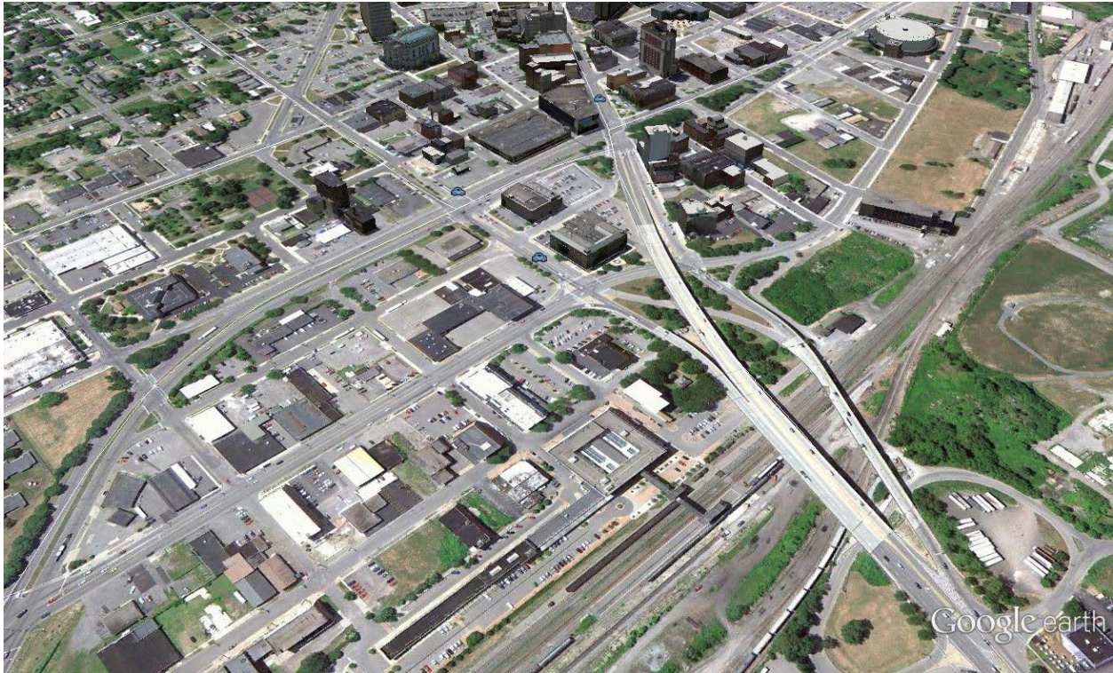
Figure 7: Utica's Union Station (center bottom), with a considerable amount of developable urban property nearby.
